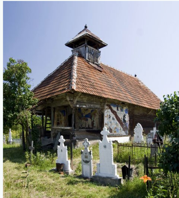
Figure 4. Wooden church from Frătesti, Gorj county.
